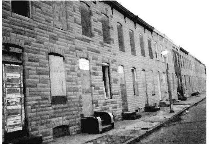
One block at a time, the buildings are coming down.
